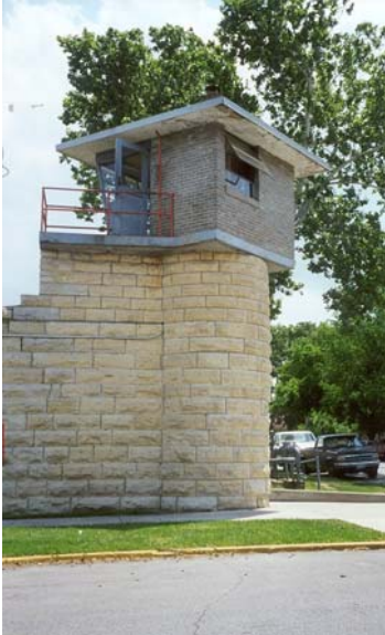
Existing Turret at Tower 2
