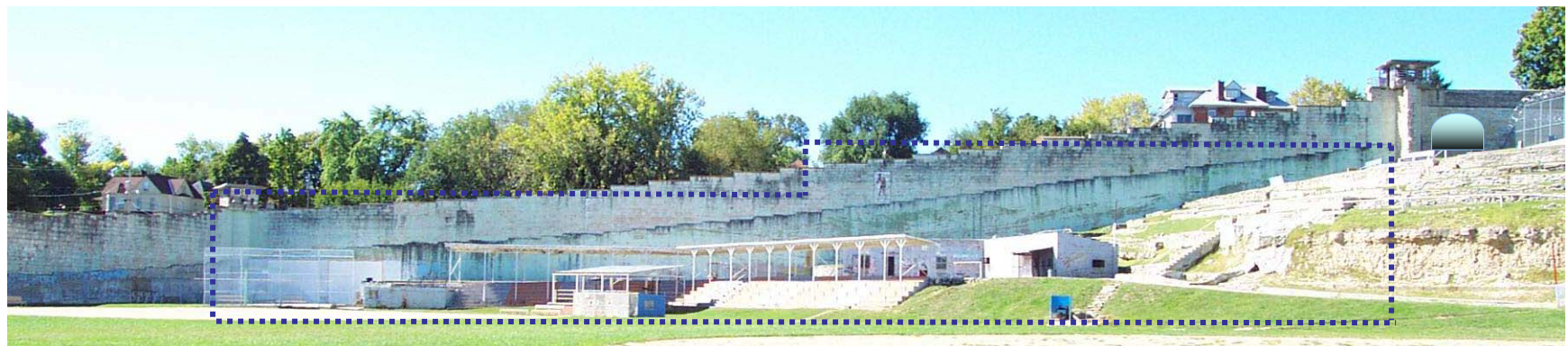
Structured Parking Profile
